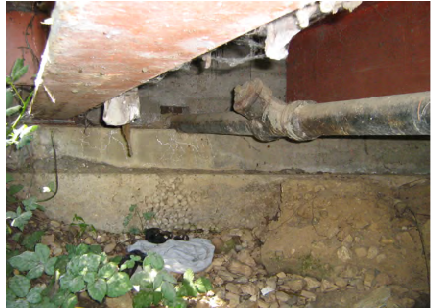
Painted steel beams below bridge. Taber Consultants photo 6/20/2006.
